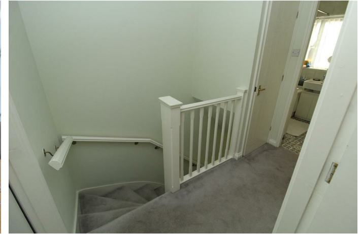
built in cupboard, access to loft space
